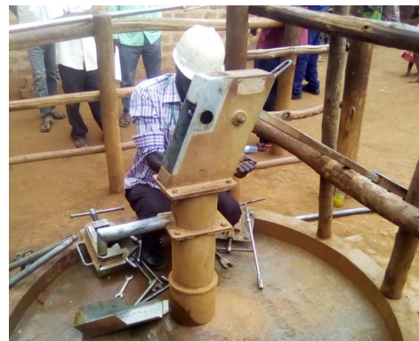
Photo 1 Repairing a Hand Pump
